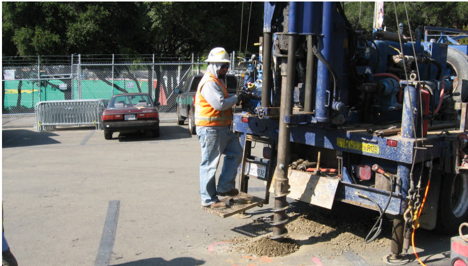
Photograph 10: View of auger drilling BL 7, facing northwest
