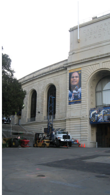
Photograph 6: View of drill rig at northwest entrance of stadium, facing east
