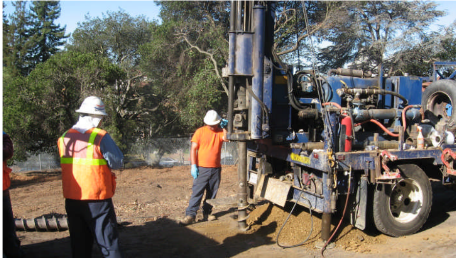
Photograph 1: View of auger drilling BL 35, facing west
