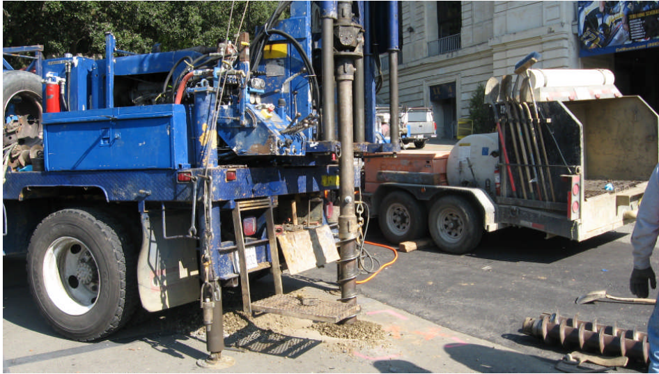
Photograph 9: View showing beginning of drilling for BL 7, facing east
